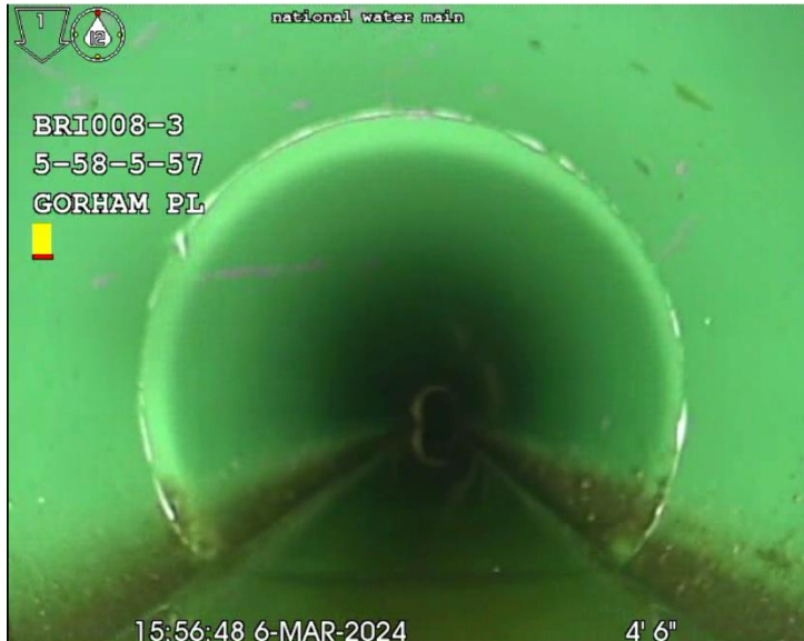
Structurally Sound Pipe
