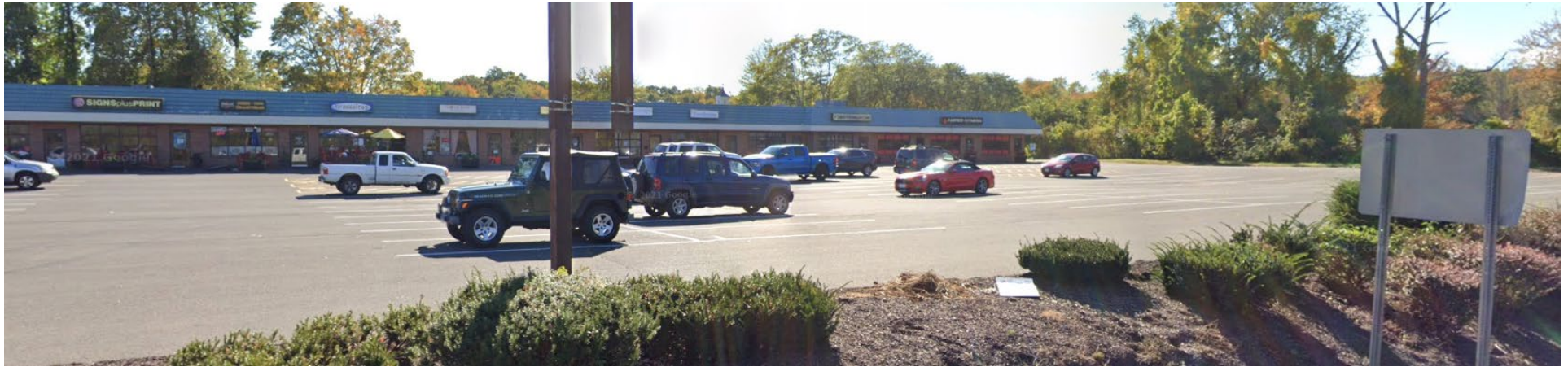
Existing Retail Plaza: Single Level, No Undulation to the Facade
