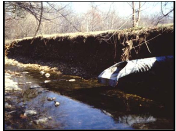
Figure 1.4.3 – Stream Channel Impacts (R.Claytor file photo)
